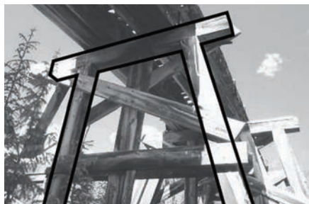
The BENT on a trestle bridge is key to giving the structure its integrity.
