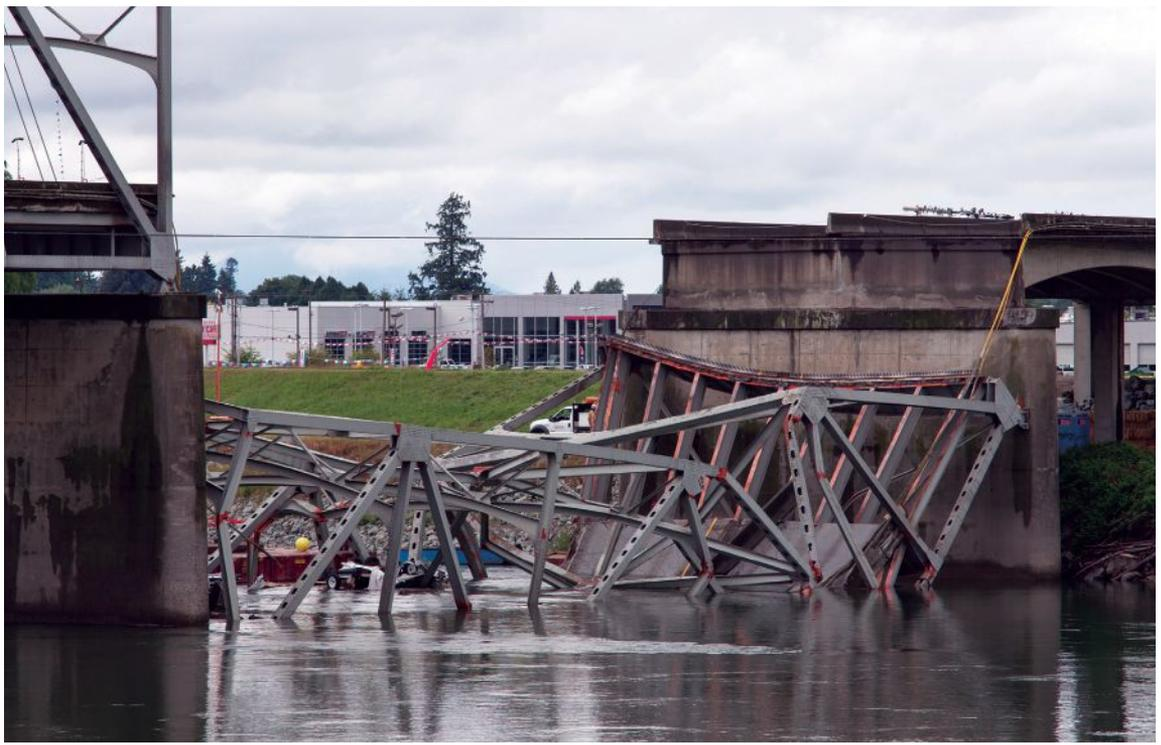
The aftermath of the 2013 Skagit River Bridge collapse in Washington. It had been classified as fracture-critical.
