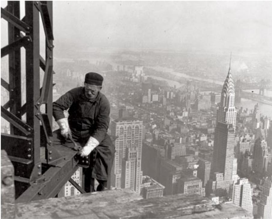
A construction worker installs girder bolts on New York City’s Empire State Building in 1931, with the Chrysler Building shown behind.
