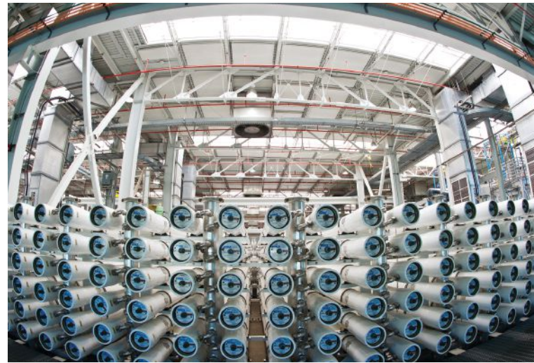
Orange County Water District manages the large groundwater basin that provides reliable, high quality groundwater to 19 municipal and special water districts that serve 2.4 million customers in north and central Orange County. Shown here, an array of reverse osmosis cartridges. Credit: Orange County Water District
