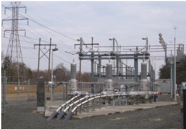
The world's first high-temperature-superconductor power transmission cable system (above) was energized in Long Island Power Authority's grid in April 2008. This system, which consists of three cables running in parallel in a four-foot-wide right of way, is capable of carrying 574 megawatts of power. The three cables shown entering the ground can carry as much power as all of the overhead lines on the far left.
