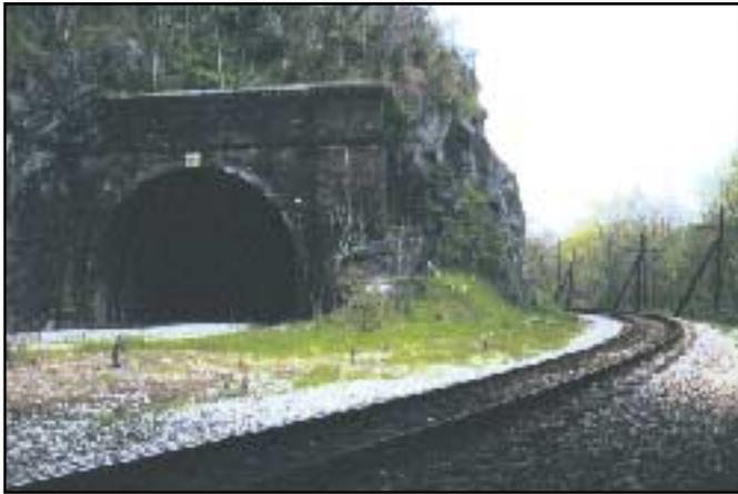
*The final insult. When the new longer and taller railway cars wouldn't fit through the old double-track tunnel at Point of Rocks, one track was moved to the center of the tunnel and the now-defunct canal filled in for the other (milepost 49).*
