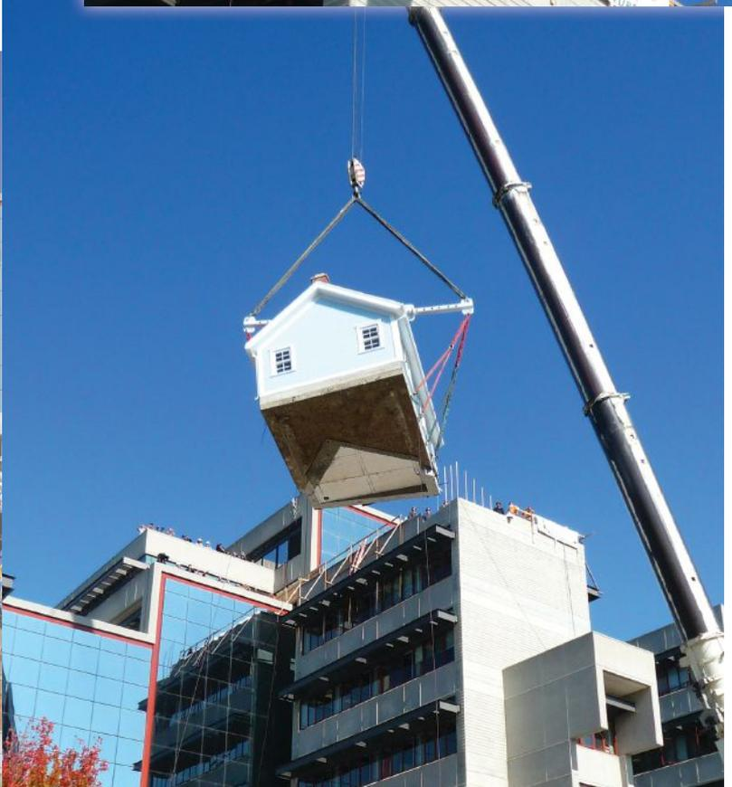
created an x-y-z coordinate system with the origin at the southwest corner of the cottage's roof. From there, the contractor was given sketches showing other points of the structure in three-dimensional space including the tops of footings, bottoms of footings, roof peak-lines, and the roof peak. The contractor then had to use story poles and string to find these points in space in order to construct the framework and foundation.
