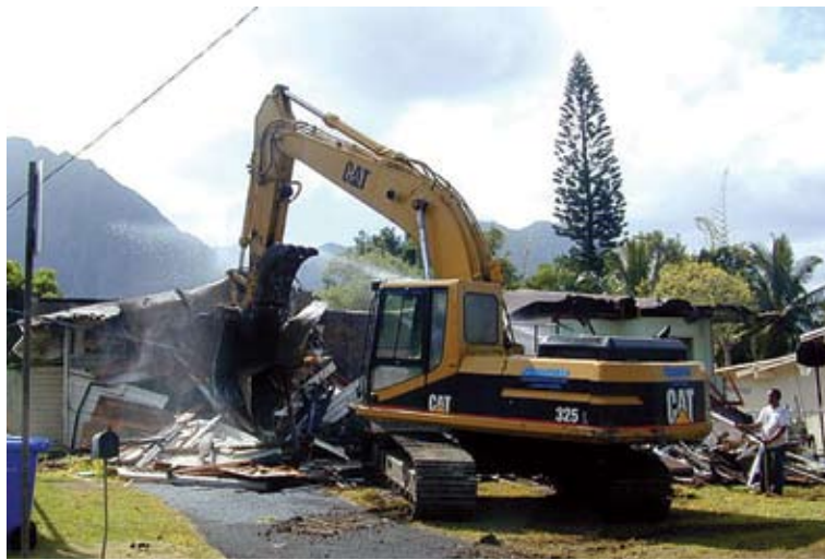
An excavator demolishes a house in Hawaii recently.
