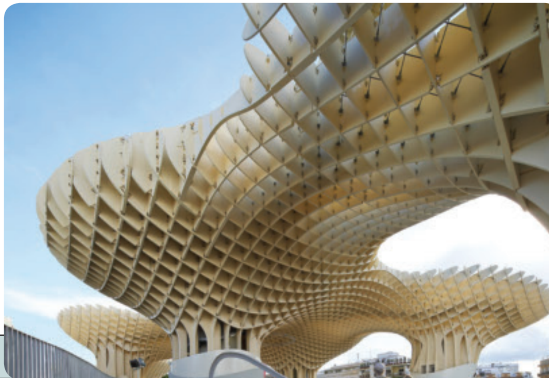
Metropol Station in Seville, Spain. Image courtesy of Arup.
