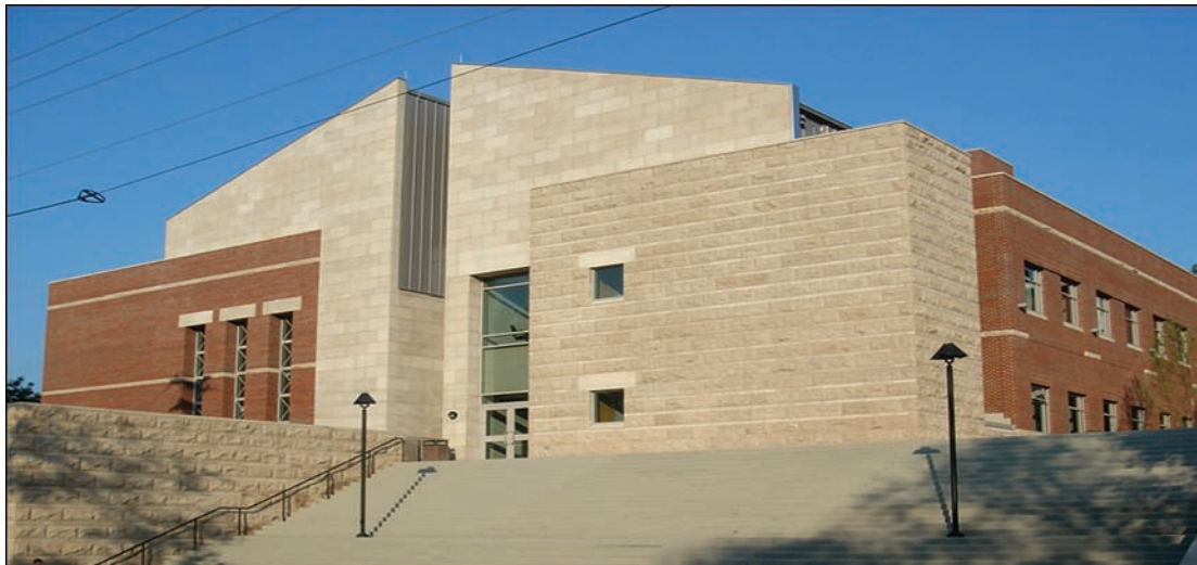
The complex for engineering and biological sciences on the WKU campus.
