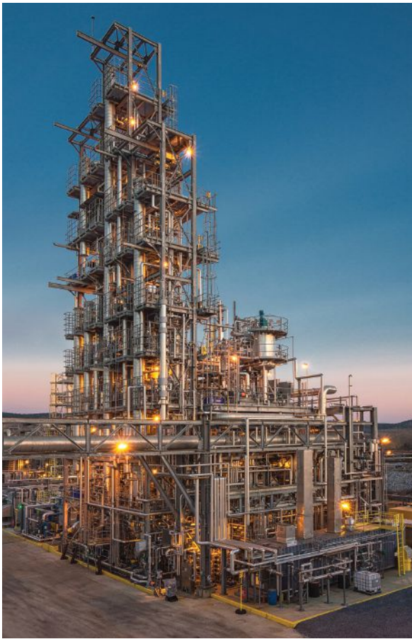
Figure 4: The U.S. Department of Energy's National Carbon Capture Center in Wilsonville, AL, has, for more than a decade, tested 60+ methods of capturing carbon dioxide from flue gases of fossil-fuel power plants as well as testing technologies for direct air capture. It is available to developers in the U.S. and other countries aiming to field pilot technologies with a goal of attaining commercial scale with net-zero greenhouse gas emissions.
