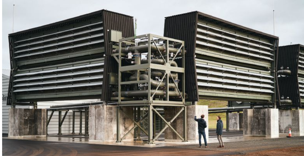
Figures 5: Beginning operation in September 2021, the Orca direct air capture (DAC) facility (above) in Iceland is powered by a nearby geothermal generating plant. Orca is constructed with eight modular units, each about the size of a shipping container, stacked two high. Each unit has a dozen giant fans (facing away from the viewer) that draw in ambient air, which passes over a sorbent filter that traps CO 2 . Once the filter is saturated, the unit heats the sorbent to the boiling point of water to release the separated CO 2 , which is piped to a connecting building. There it is mixed with water (27 tons of water per ton of CO 2 ); the resulting carbonated water then is piped about a quarter mile where it is injected deep into the Earth. Underground, it chemically reacts with Iceland’s abundant basalts to produce carbonate minerals (left), permanently trapping the CO 2 over about two years. Credit: Climeworks
