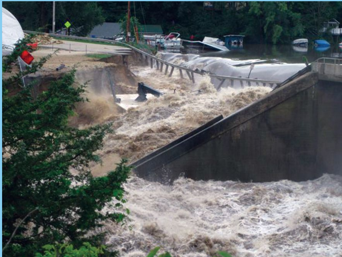
The 59-foot-high Lake Delhi Dam in Iowa failed in 2010 when it was overtopped during record rainfall. A 2009 inspection of the 80-year-old dam had revealed one of three spillway gates was inoperable; also, a strengthening concrete core wall did not reach the embankment’s maximum height, allowing seepage to weaken the dam. Emergency responders evacuated downstream residents fast enough that no lives were lost. PHOTO: Iowa Department of Natural Resources.
