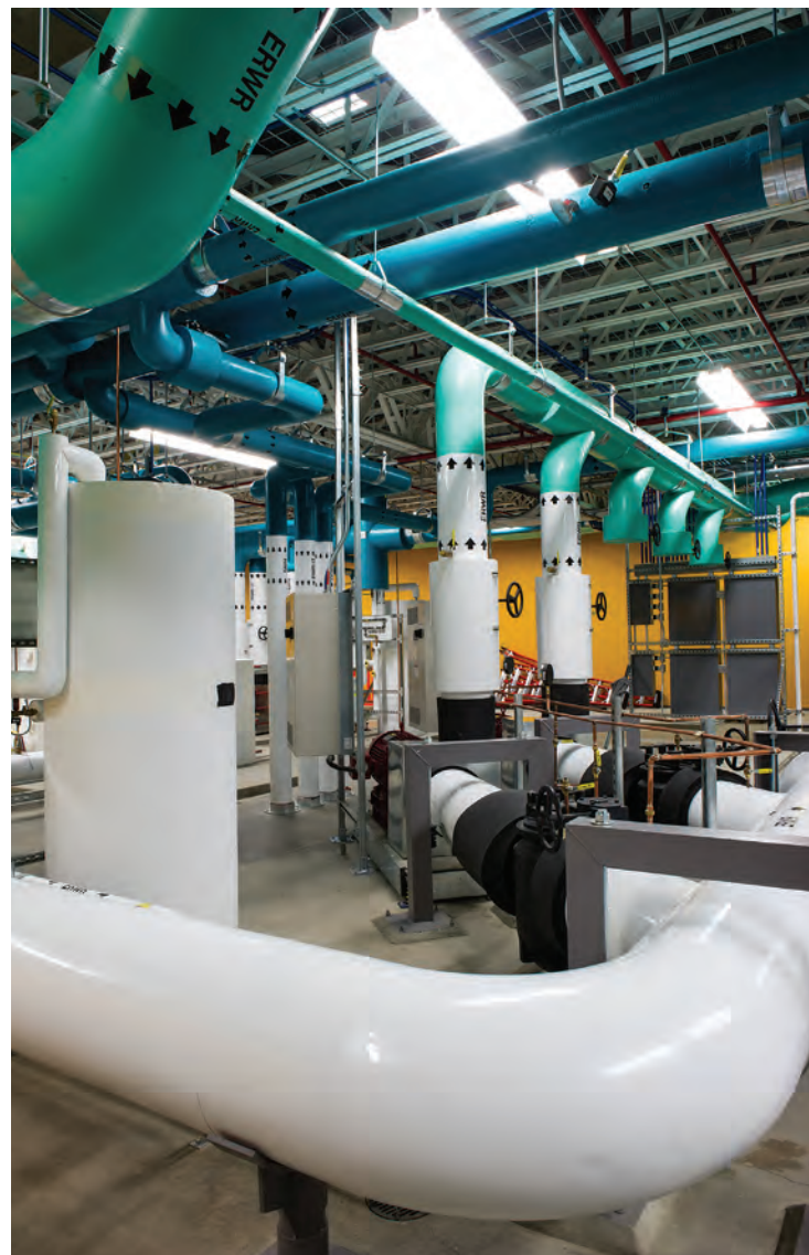
ABOVE: Steve Hammond, director of the computational science center at the NREL, stands in front of computer racks in the high performance computing data center. BELOW: Pipes circulate water beneath the high performance computing data center. Photos: Dennis Schroeder/NREL .
