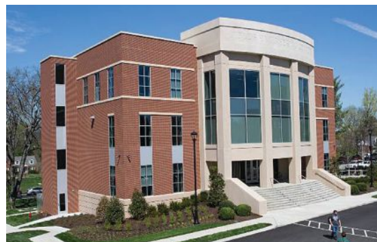
Top Image: Driftmier Engineering Center. Bottom Image: Fields Engineering Center.
