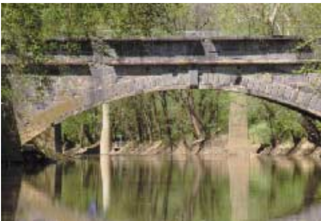
Three eras of transportation: the aqueduct is from the canal; the rectangular pillars are from the railroad (now also a hike/bike path); the round pillar is the present highway bridge (milepost 116).
