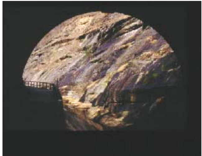
Paw Paw tunnel — looking out of the tunnel into the cut (milepost 155).
