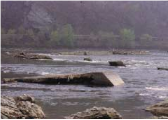
Ruins of dam #3, damaged in the flood of 1924 that closed the canal (milepost 64).
