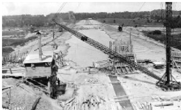
General view of the partially completed Englewood Dam, March 25, 1921, looks east along the dam’s centerline from near the spillway. The largest of the five dams, it stretches 6,400 feet across the Stillwater River. Source: Miami Conservancy District
