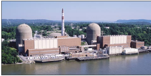
Figure 8 (left) Indian Point, located 35 miles north of New York City, has two operating reactors—far left and right in photograph—and a mothballed unit (center). Activists have argued for its shutdown for more than 30 years.
