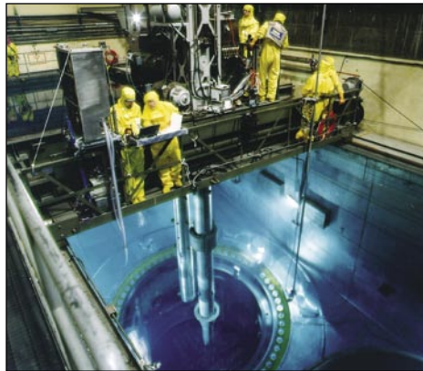
Figure 4 (above) Refueling the reactor at Arkansas Nuclear One in Russellville, AR.
