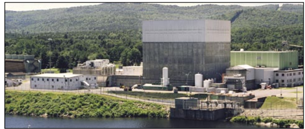
Figure 9 Entergy’s Yankee nuclear plant generates about one-third of Vermont’s electricity. The unit has proven very profitable since the runup in natural gas costs.
